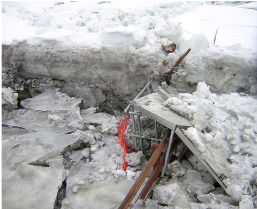
Photo 2: Disabled access fishing platform damaged by ice in 2007.
