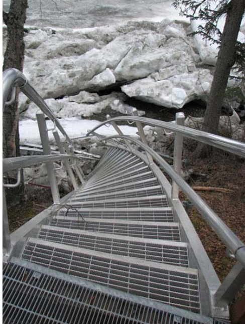
Photo 1: Staircase at the Kenai River Center damaged by ice in 2007.
